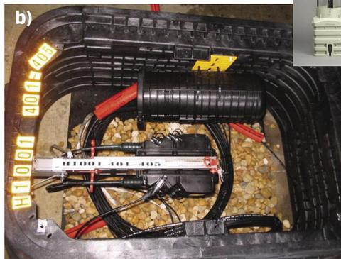
**Photo 2.** There are several factors to consider when deciding between an above-ground pedestal NAP (a) and below-ground handhole (b) configuration.
