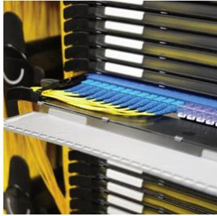
Corning's Centrix platform is a high-density, modular, and scalable fibre management solution, that can be used in LAN backbone applications where there is a large number of fibre connections. Airports, large campuses, or hospitals are examples. The system supports a modular "build-as-you-grow" approach, using cassettes and different types of housings or frames. The modular cassette contains up to either 24 SC or 36 LC connector adapters and can be tailored to include a splitter.
